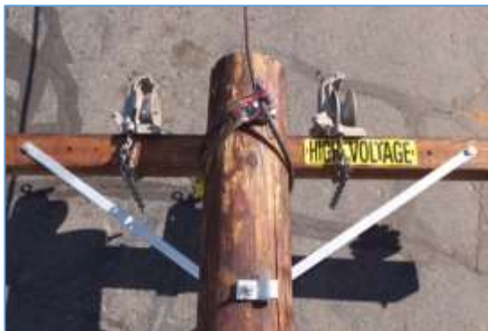
Figure 25: Incorrect, Shackle Upside Down
