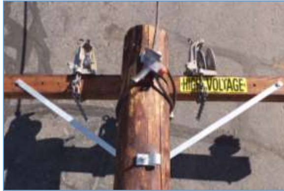
Figure 27: Correct Cable Saver Installation
