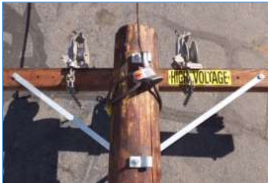
Figure 28: Incorrect, Cable Saver Upside Down
