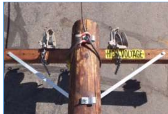
Figure 26: Incorrect, Screw-Pin Eye into Pole
