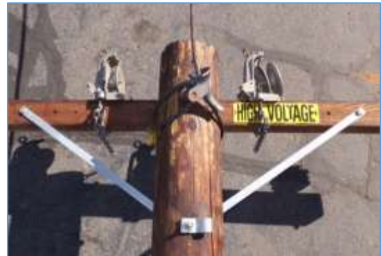
Figure 29: Incorrect, Screw-Pin Eye Against Pole
